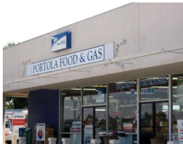
The Portola Food & Gas convenience store has used CoolTrol Cooler Control Systems since March 2006.
