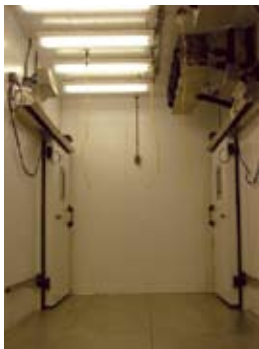
Cold Storage Room
