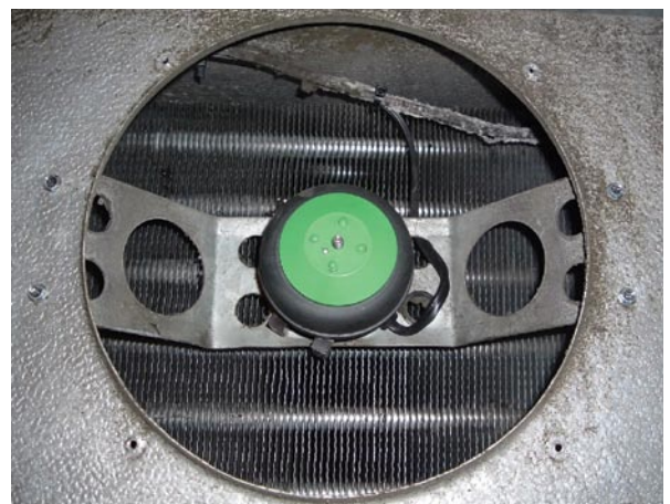
The picture above shows the NRM SSC 2 motor installed in Walk-in Cooler Evaporator Coil (before the blade is installed).
