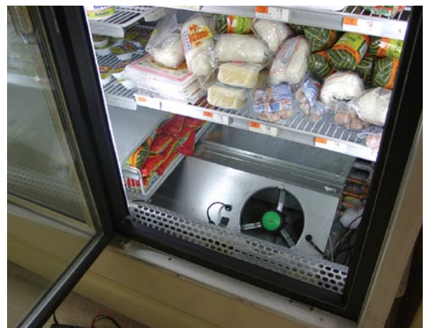
Here the NRM SSC 2 motor is installed in a frozen case (before the blade is installed).
